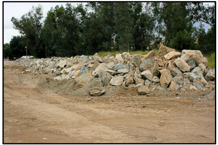
MORE THAN A ROCK PILE: These boulders will soon line Coldwater Creek to prevent flooding and erosion.
