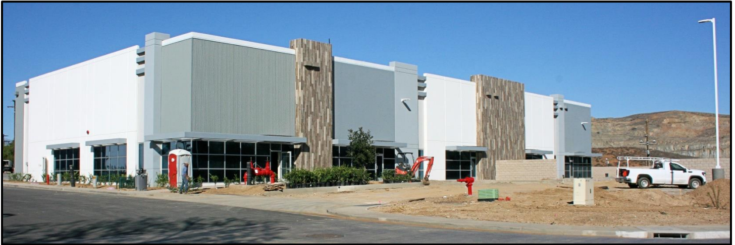
LAKE MATHEWS SHERIFF'S STATION: The county is leasing a 20,000-square-foot building in the new Latitude Business Park in the city of Corona that will provide Sheriff's services to eight unincorporated communities, including Temescal Valley.
